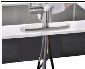
1. Place all the hoses into the sink hole.
