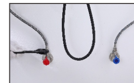
4.Connect the water supply hoses to the angle valves.
