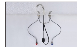
6.The installation is complete. Turn on the handle to check for any leaks.
